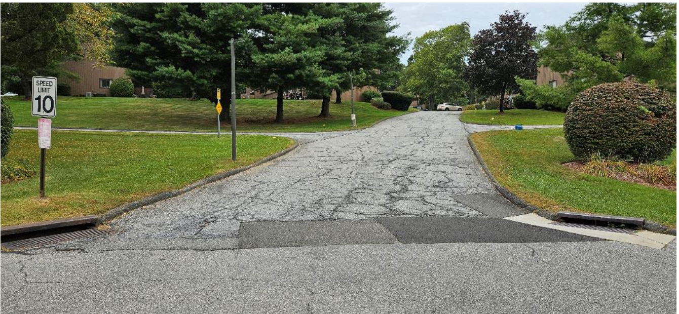
Amherst Road within development looking northwest towards a private driveway
